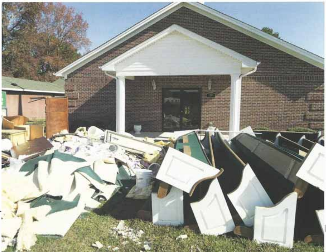
As one of the first steps in recovering following a damaging storm, buildings are gutted of their contents to be dried out and renovated.
